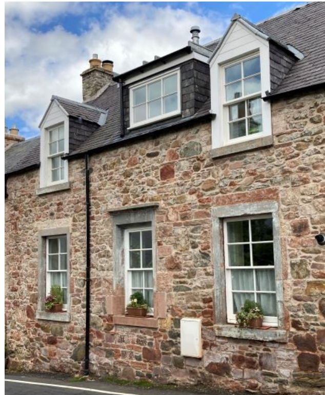
Fig. 56 To the left and right, traditionally-scaled and detailed dormers align with the windows below. This format could be followed. To the centre, a later box dormer of non-traditional design and poorly-aligned with windows below. This format would not be acceptable where visible in the streetscene.
