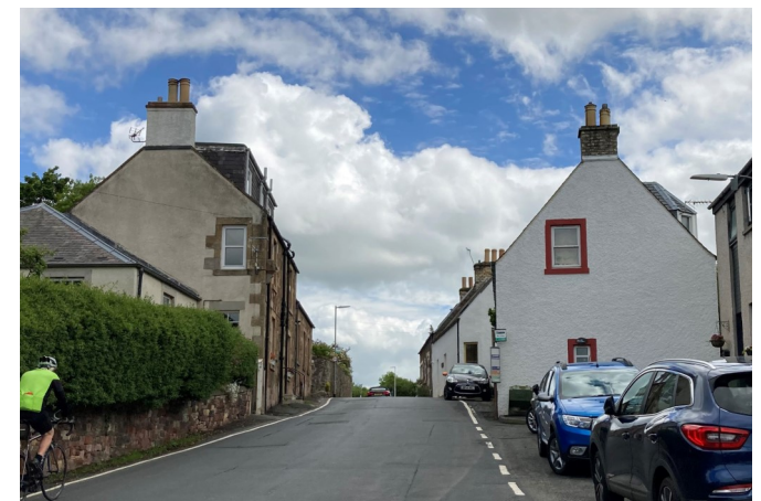
Fig. 25 (bottom): Gable end elevations are prominent in the conservation area. They tend to incorporate chimney stacks and some limited fenestration.
